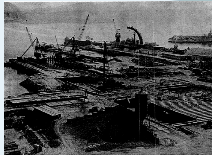
O.N. 47374: Marine Lift, Simonstown - A recent view of the site by courtesy of the S.A. Navy.
